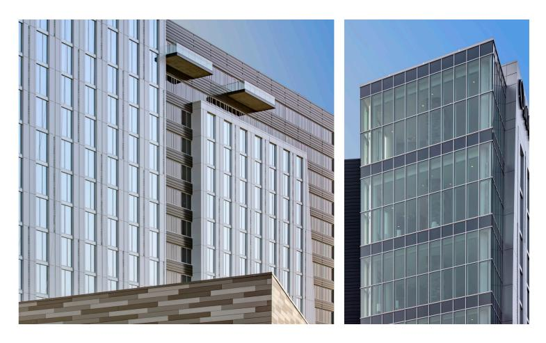
d 5mm) thermal break ard 6" (152.4mm) system depth and 1-3/16" (30.2mm) tape glazed
